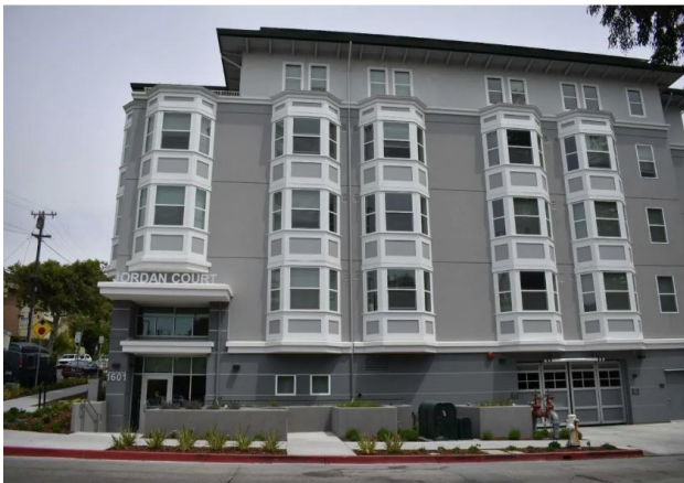
Photo credit to berkeleyside—Jordan Court Affordable Housing
